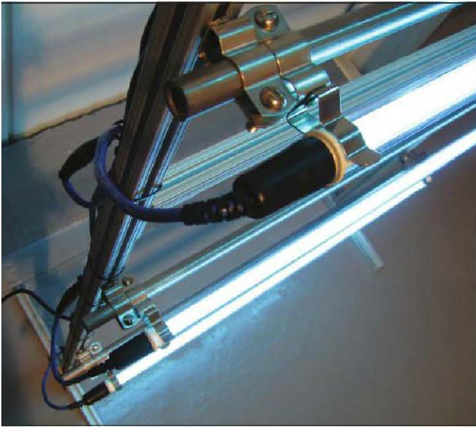
A tubular rack UVGI system is a quick and easy method of installing UV lights as a retrofit or new installation in any brand and size of commercial HVAC equipment. The installation kit uses common electrical conduit and brackets so maintenance departments and contractors can custom build a system into an AHU.
