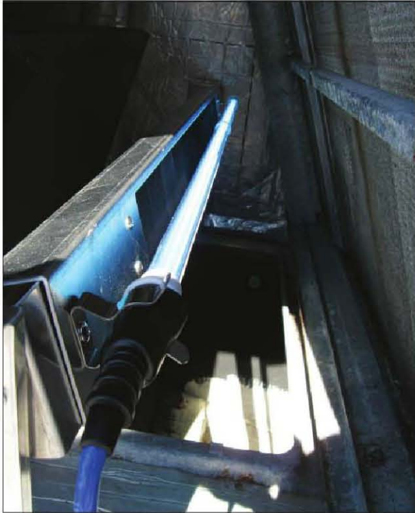
This photo shows an air-handler installation that uses a combination of UVGI, gas-phase air purification, and PCO in one unit for total air purification.
